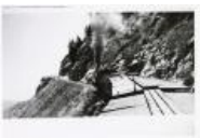
Uintah locomotive climbing 7.5% grade on Baxter Pass. (1987.39.5)
