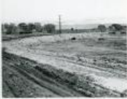
Gunnison Bridge and dike (1983.63.9)
