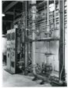
Pilot Plant - Grand Junction (1983.63.131)
