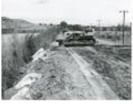
CAT bulldozer pushing riprap into river bank (1983.63.7)
