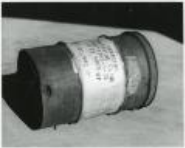
This corroded drum requires only a light blow with a screwdriver to pierce the metal and tear (1983.63.161)
