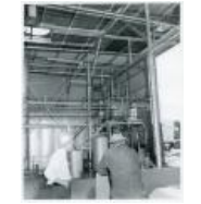
Inside new boiler house AEC Compound (26 Sep 1956) (1983.63.115)
