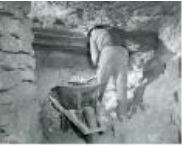
Hand loading ore into a wheelbarrow (1983.63.73)
