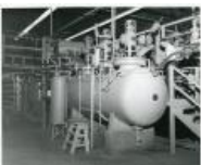
Alkaline Leach Autoclave - Pilot Plant, Grand Junction (1983.63.136)
