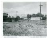
Getting sampling plant expansion slab area ready for pour (1983.63.146)
