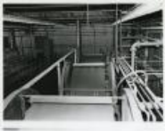
Pilot Plant - Grand Junction (1983.63.132)
