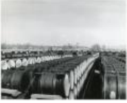
Vanadium storage closeup view looking Northwest (1983.63.158)
