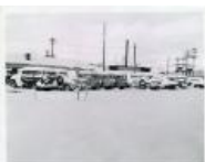
Snow storm at AEC Compound Grd. Jct. Cars covered (1983.63.119)
