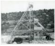
Steel headframe and ore bins at Colorado Plateau. Vertical Shaft operations. (1983.63.176)
