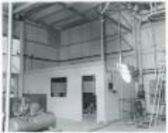
New boiler house building (1956) (1983.63.113)
