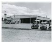
AEC Sampling Plant Expansion site (23 Jul 1956) (1983.63.141)
