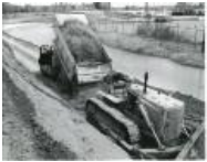
Dump truck unloading fill on dike (1983.63.4)
