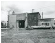
AEC Heating Plant (May 1957) (1983.63.125)
