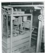
Pilot Plant - Grand Junction (1983.63.135)
