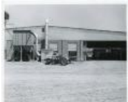
AEC Sampling Plant Expansion site (23 Jul 1956) (1983.63.140)
