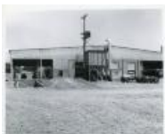
AEC Sampling Plant Expansion site (23 Jul 1956) (1983.63.142)
