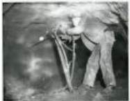
Drilling blast holes in a Colorado Plateau uranium mine. Miner is using a Jack-let type percussion drill. (1983.63.180)
