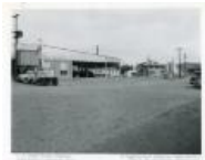
AEC Sampling Plant Expansion site (23 Jul 1956) (1983.63.143)
