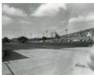
Grand Junction Compound paving parking lot (9 July 1957) [Duplicate] (1983.63.108)
