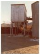
Silo with drums in background (1983.63.231)
