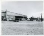
AEC Sampling Plant Expansion site (23 Jul 1956) (1983.63.139)
