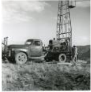
Johnson and Youran Drilling Co., Naturita, CO Drilling rig (1983.63.96)
