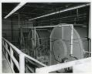
Pilot Plant - Grand Junction (1983.63.133)
