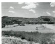
Grand Junction Compound parking lot prior to black topping (18 June 1957) [Duplicate] [Duplicate] [Duplicate] (1983.63.105)
