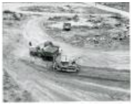
Loading fill for dike across road from AEC compound (1983.63.11)
