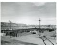
Overall view of vanadium storage looking Northwest (18 Feb 1958) (1983.63.156)
