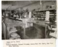
Photo of the Interior of the J.W. Hugus and Co. Store (1979.23.149)
