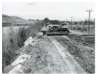
CAT bulldozer pushing riprap into river bank (1983.63.7)
