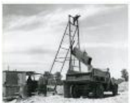
Headframe and skip hoist at small uranium mine. This is an inclined shaft mine. (1983.63.187)
