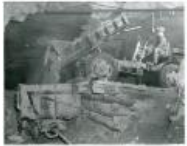
Underground dumping ore from diesel dump truck into Granby type car (1983.63.183)
