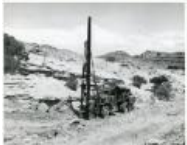
Exploratory drilling for uranium with truck-mounted pneumatic percussion drill (1983.63.189)
