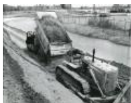
Dump truck unloading fill on dike (1983.63.4)
