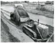
Dump truck unloading fill on dike (1983.63.4)
