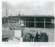
Starting construction SS Sampling plant expansion south dock showing new concrete slab (4 Sep 1956) (1983.63.145)
