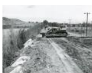
CAT bulldozer pushing riprap into river bank (1983.63.7)
