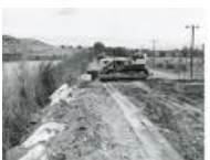
CAT bulldozer pushing riprap into river bank (1983.63.7)
