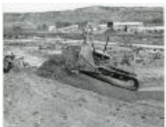
CAT Bulldozer pushing up fill across road (1983.63.12)
