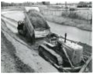
Dump truck unloading fill on dike (1983.63.4)
